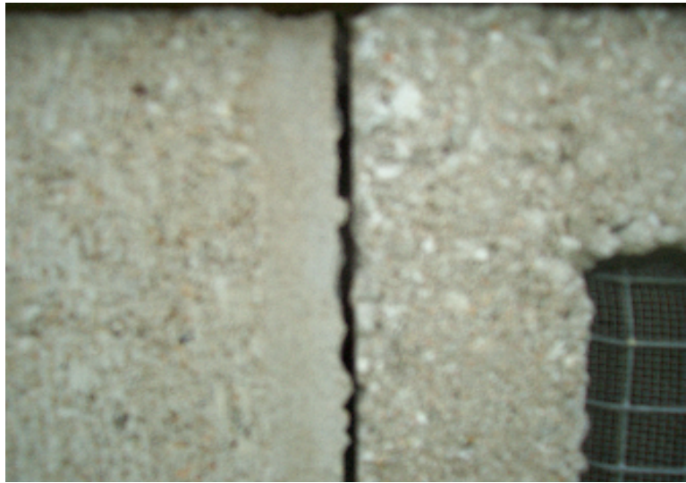
FOUNDATION MORTAR CRACK.
