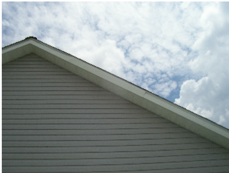
LOOSE SOFFIT WEST.
